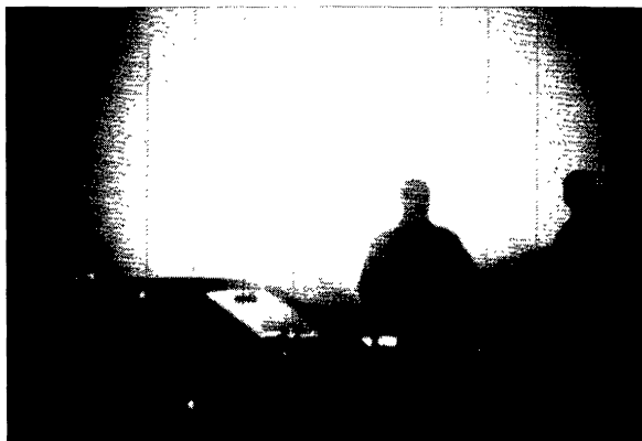
A poorly-mounted, over-bright 'security' light at a previously dark New Forest location. By concealing what is behind it, the light defeats the purpose for which it was installed. (Photo: Bob Mizon)
