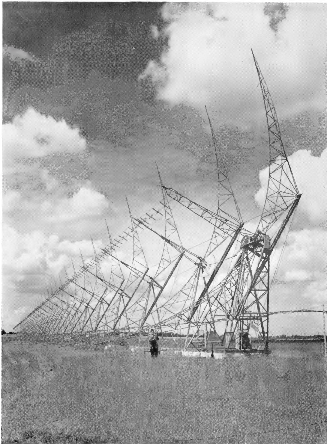
The long fixed element of the radio star interferometer.
