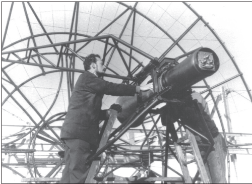
Figure 8: Marcel Parise adjusting the focal system for 21cm.
