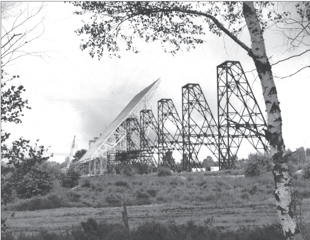
Figure 9: The fully-tiltable mirror during construction.
