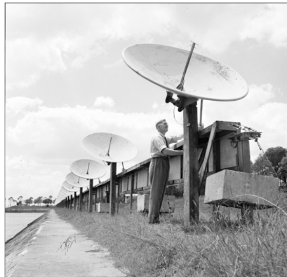
Figure 8: 'Chris' Christiansen and his 32-element East-West 1,420 MHz solar grating array at Potts Hill, Sydney (courtesy: ATNF Historical Photographic Archive).
